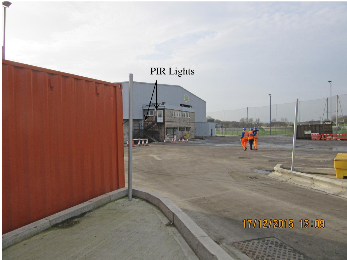
Figure 2 : Looking south west towards the MBF buildings northern elevation shows the PIR lights on the Welfare building (white circles)
