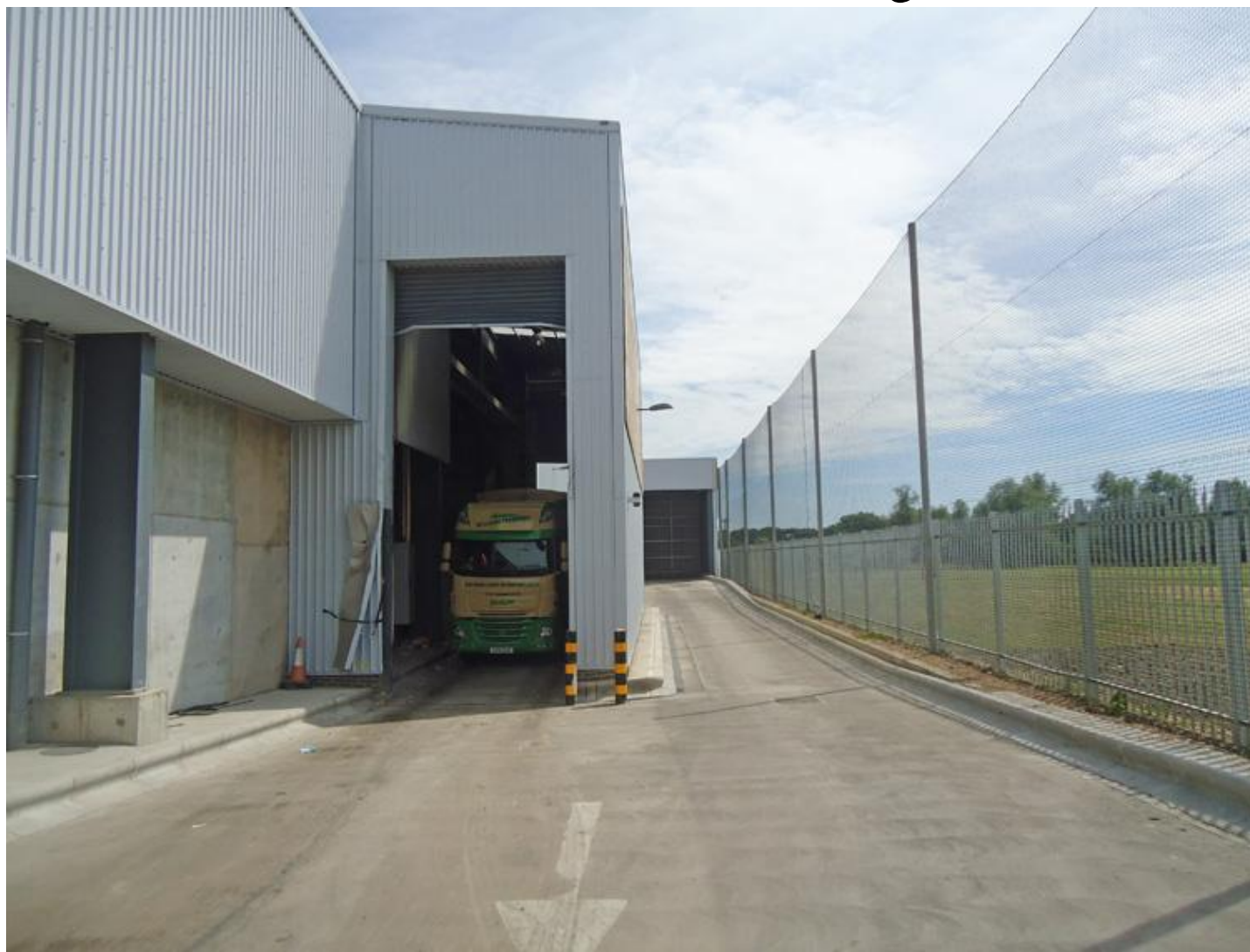
Figure 3 : Looking south towards southern boundary showing the Estilo HOLOLux with Flat Glass Wall mounted at 6 metres light fixture
